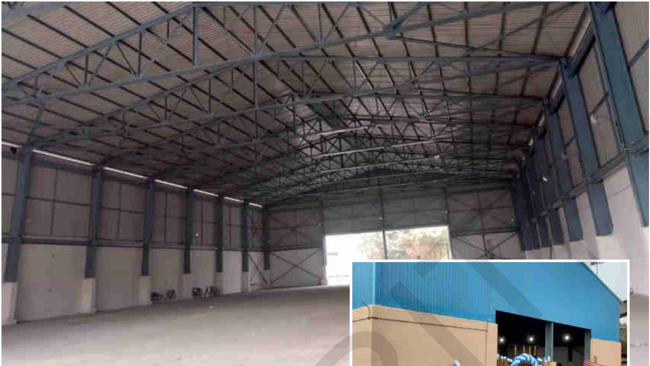
Extension of Industrial Campus OF Flender Drives Private Limited Completed
